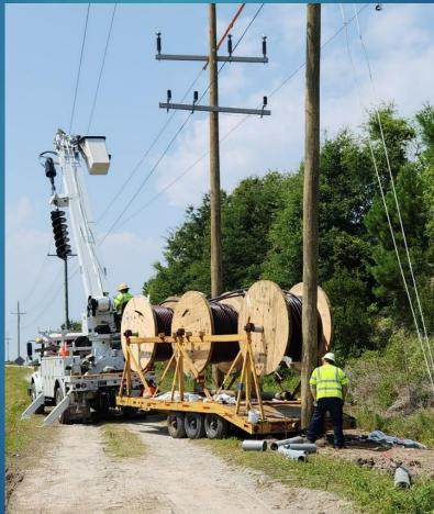
The subcontractor hired by Duke Energy to bore and place the conduit pipes for the relocation of the utilities has finished boring and are pulling the conduit pipes through. Once they are finished, Duke Energy will come in and run the wires through the conduit pipes
