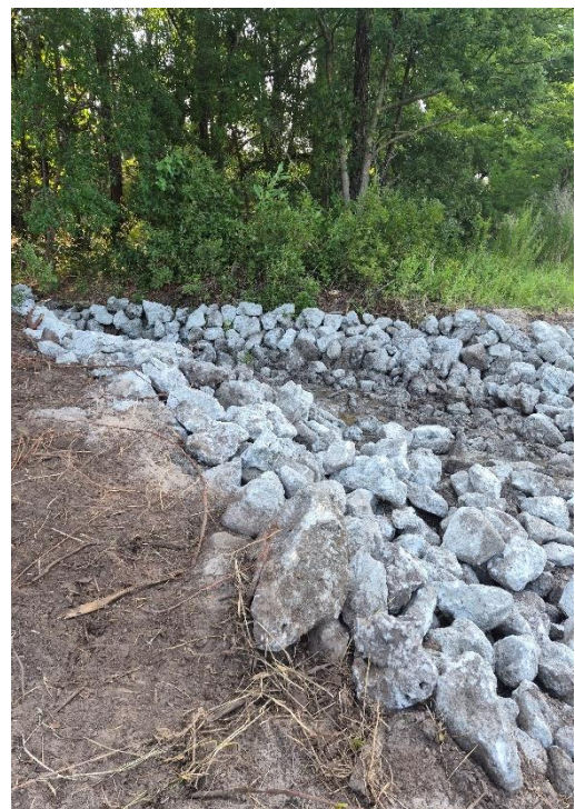
North Shore Dr. Project 2 Rip-Rap Discharge Apron
