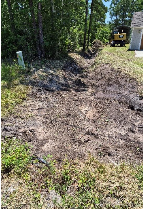
North Shore Drive Primary Ditch Rehabilitation
