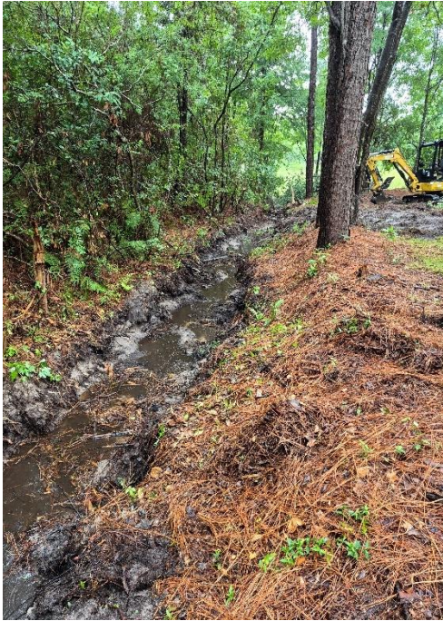
North Shore Dr. Project 2 Ditch Upgrades/Repair
