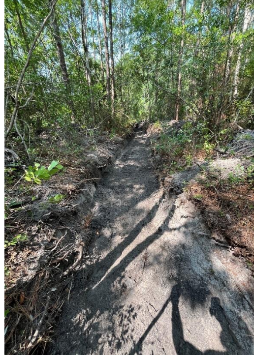
Filmore Road Ditch Clearing and Re-Shaping
