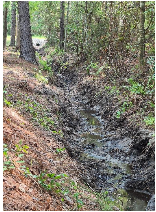
North Shore Dr. Project 2 Ditch Upgrades/Repair
