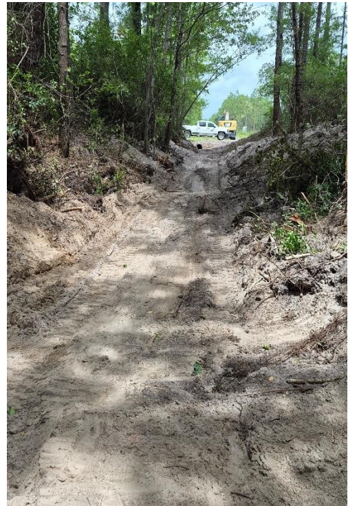
Primary Drainage Ditch Upgrades Clearing and Re-Shaping
