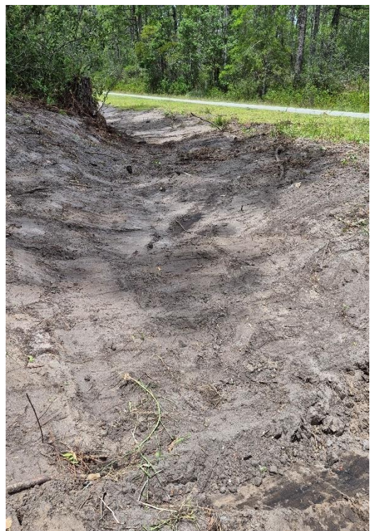
Primary Ditch Upgrades Swale/Ditch Re-Shaping
