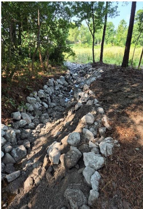
North Shore Dr. Project 2 Rip-Rap Channel/Bank Protection
