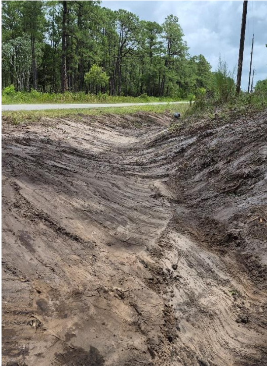
Primary Ditch Upgrades Swale/Ditch Re-Shaping
