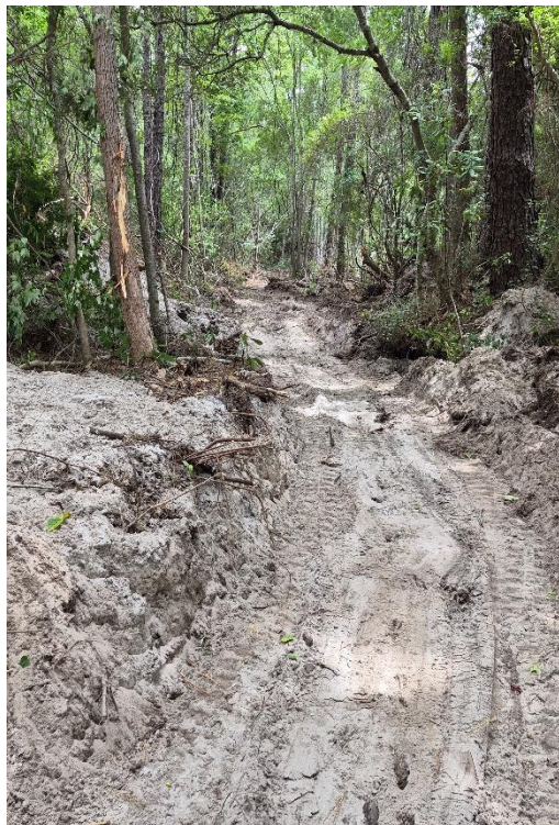
Primary Ditch Upgrades Clearing and Re-Shaping
