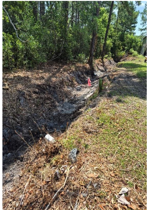
North Shore Drive Primary Ditch Rehabilitation
