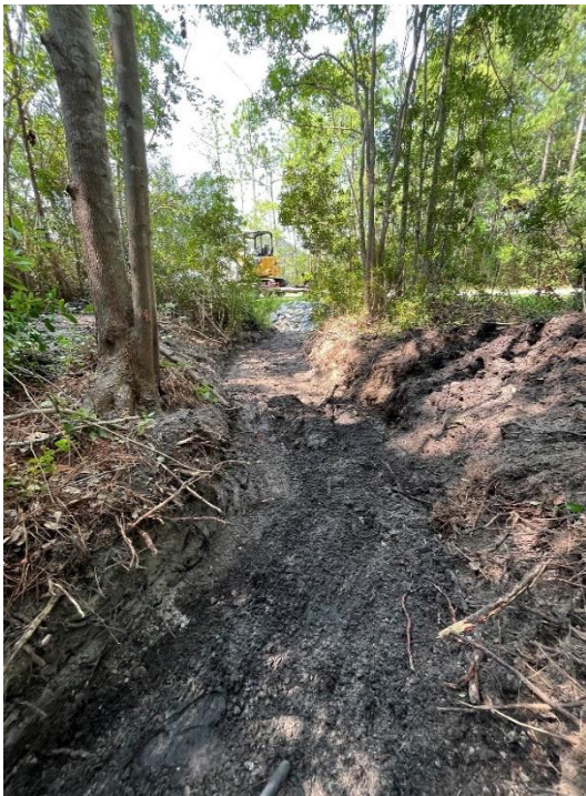
Filmore Ditch Upgrades Clearing and Re-Shaping
