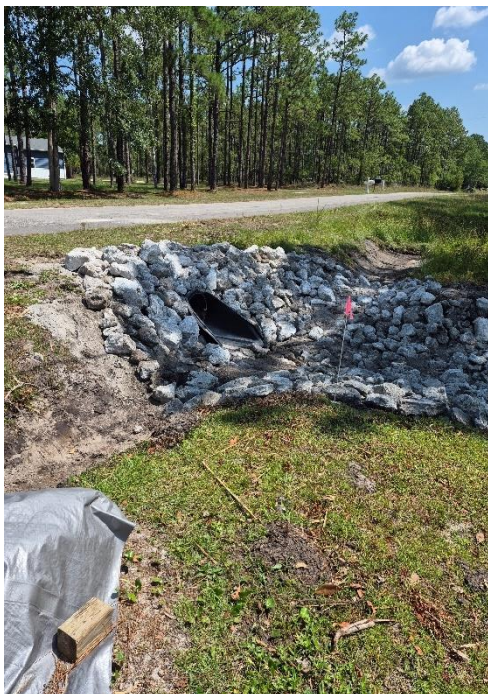
North Shore Drive Flared End Install w/Rip-Rap Protection
