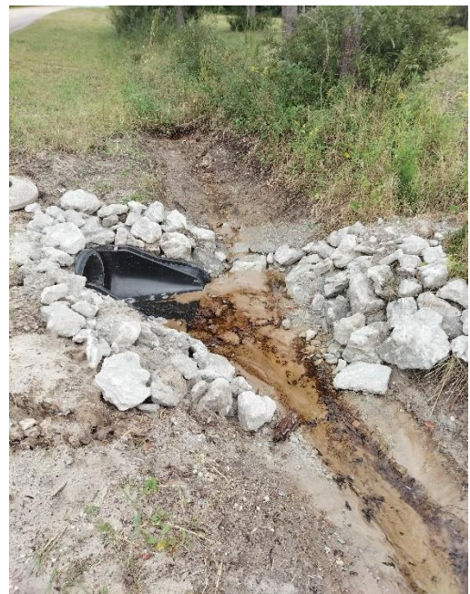
New Pipe Repair w/Flared End Section and Rip-Rap Protection
