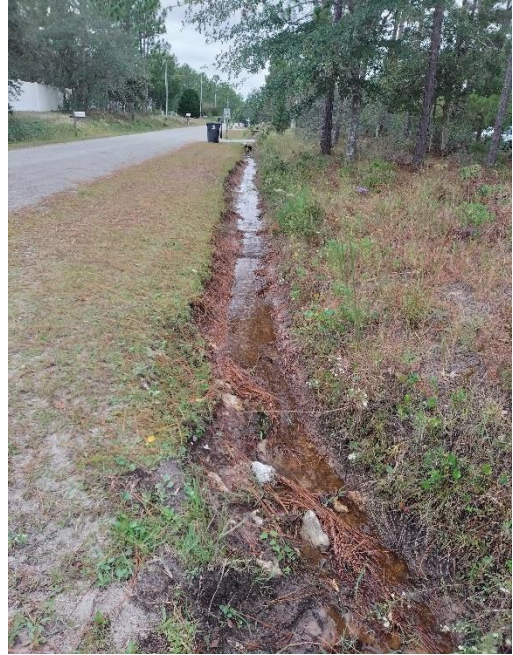
Ditch Cleaned and Shaped (typical)
