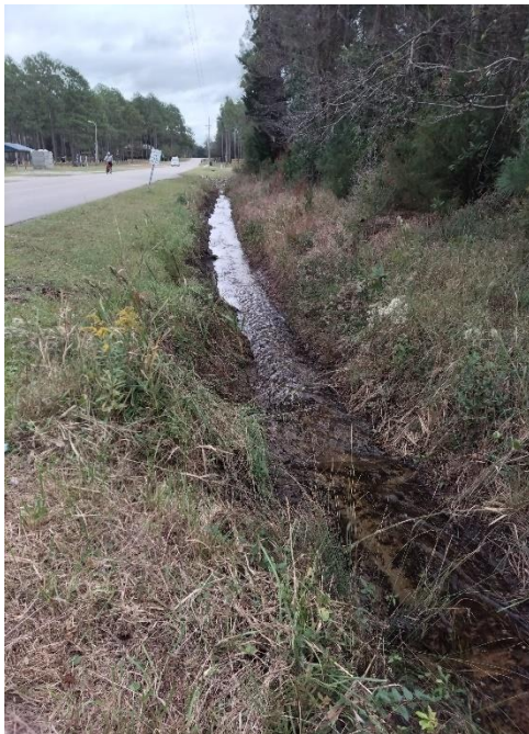
Recently Cleaned and Reshaped Ditch Unobstructed Flow
