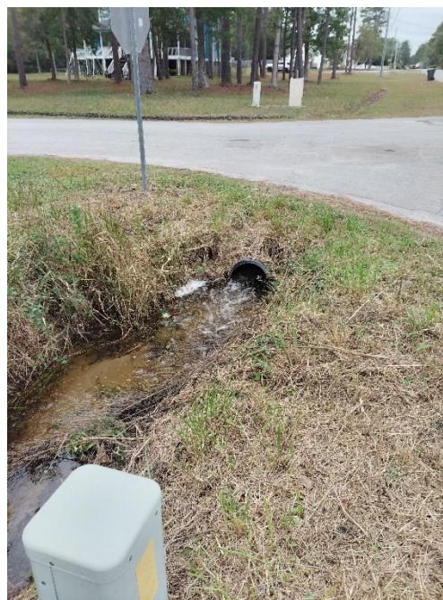
Cleaned and Reshaped Ditches Free Unobstructed Flow
