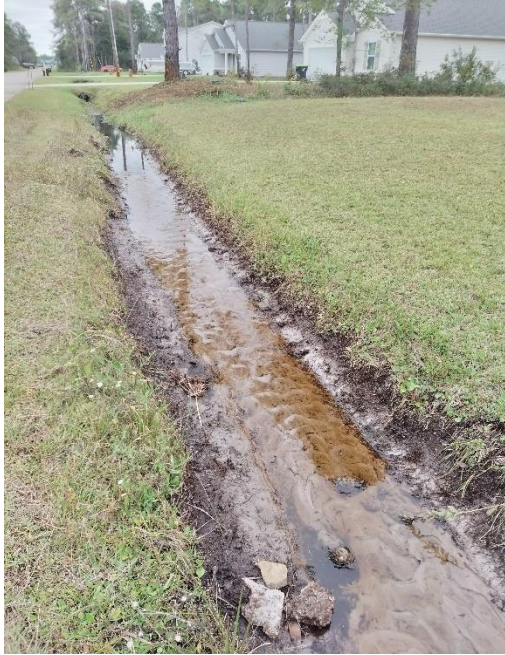
Ditch Cleaned and Shaped (typical)
