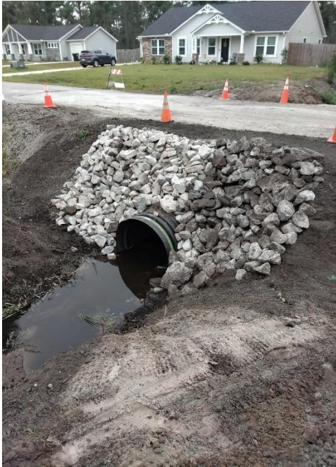
Golf View Pipe Install w/Rip-Rap Protection (Upstream)
