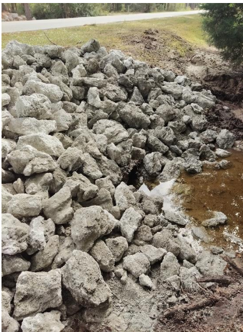
Pipe Culvert Restoration w/Rip-Rap Protection (Upstream)
