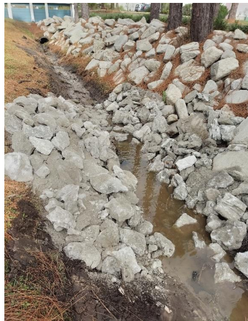
Pipe Culvert Restoration w/Rip-Rap Protection (Downstream)
