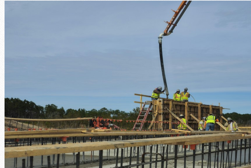
Pouring The Upper Dam Spillway #2 Outlet Wall
