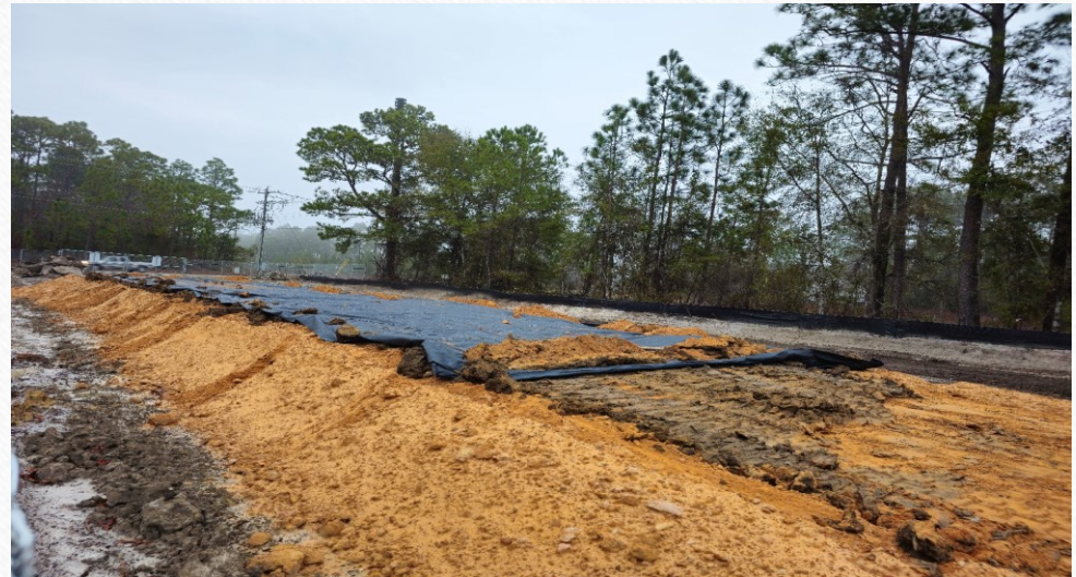
Sanford Dam Clay Core Test Panel
