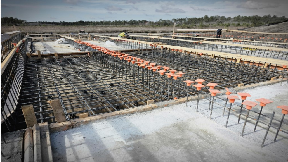
Upper Dam Spillway Floor
