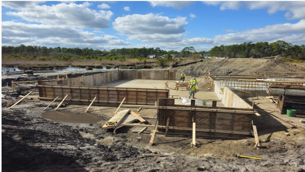
Sanford Dam Spillway Forms
