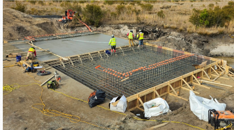
Concrete Crew Pouring the Upper Dam Outlet Base
