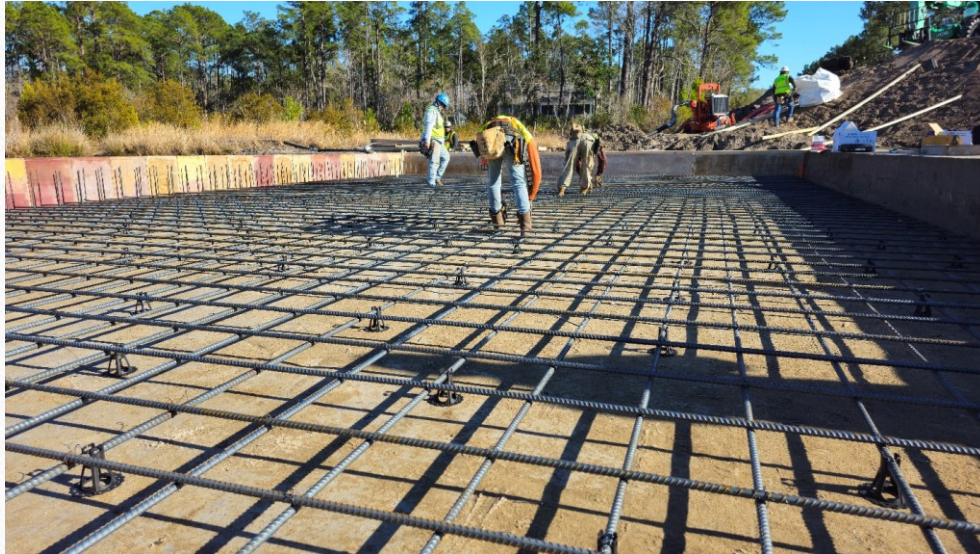
Concrete Crew Tying Steel for Upper Dam Outlet Base Slab
