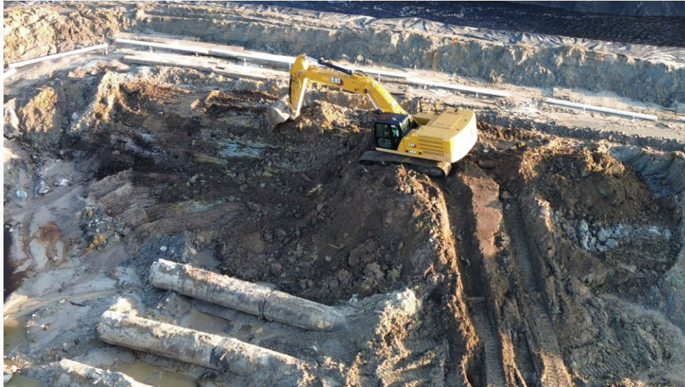
Excavating Unsuitable Spoil
