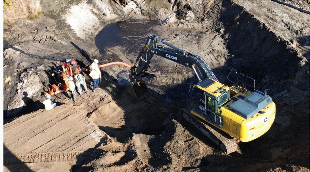
Filling/ Compacting The Upper Dam Scour Area Fill
