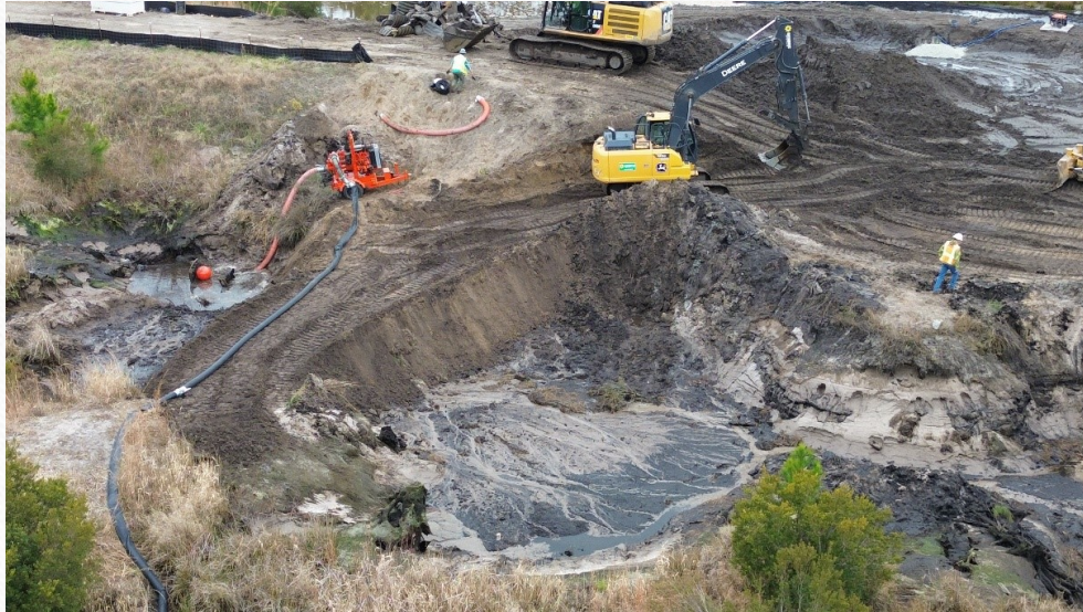
2 nd Diesel De-Watering Pump at the Upper Dam
