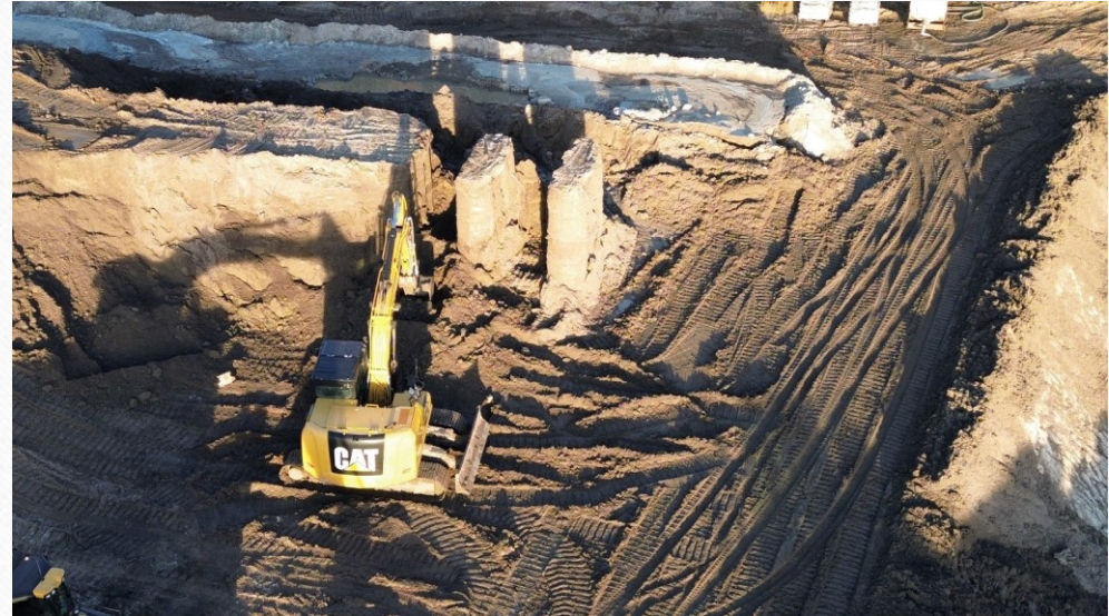
Excavating MIP Test Panels For Core Samples
