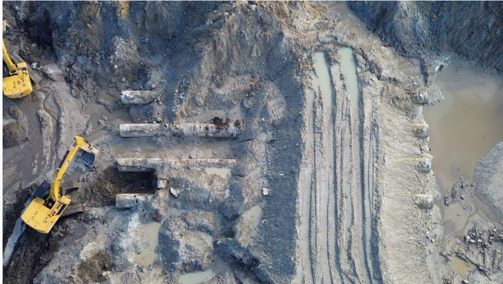
Excavating the Spillway Base
