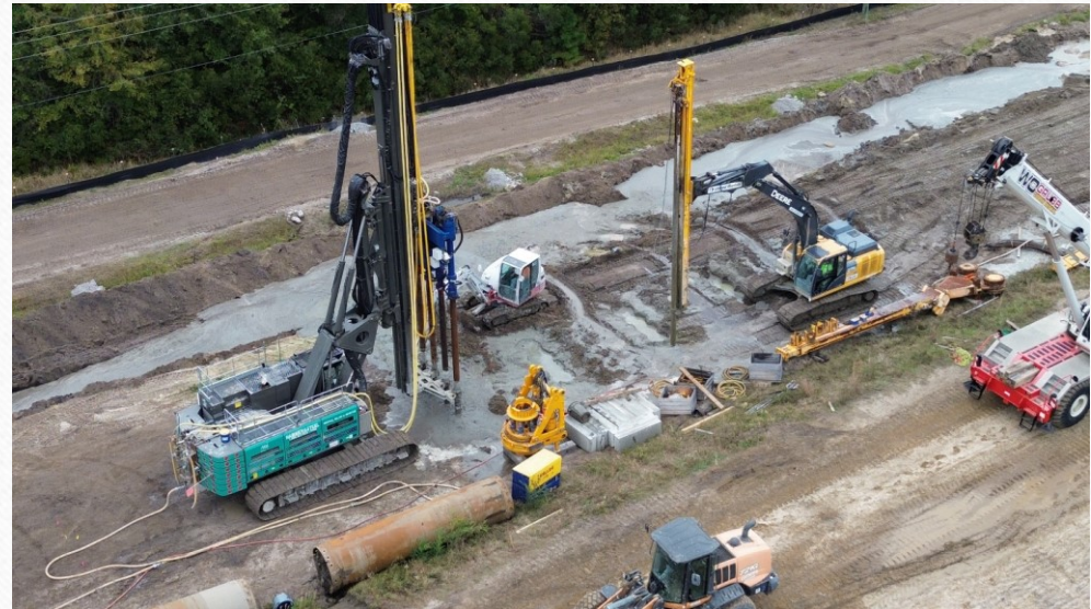
MIP Drill Installing Test Panel on Platform
