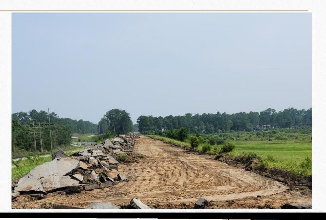
Stripping topsoil and rip rap on the Sanford Dam face
