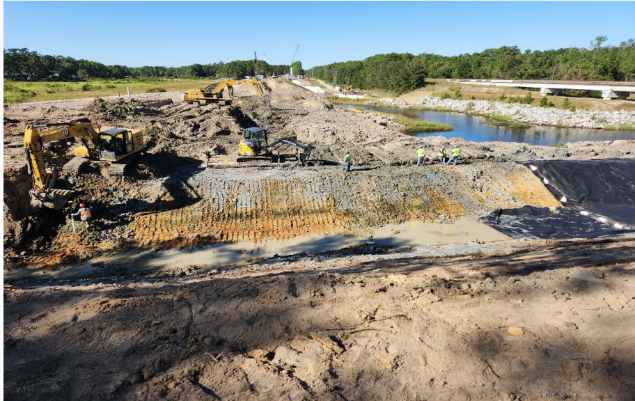
Excavating Bypass Canal
