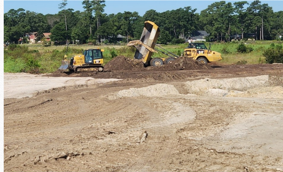
Extending Coffer Dam Base
