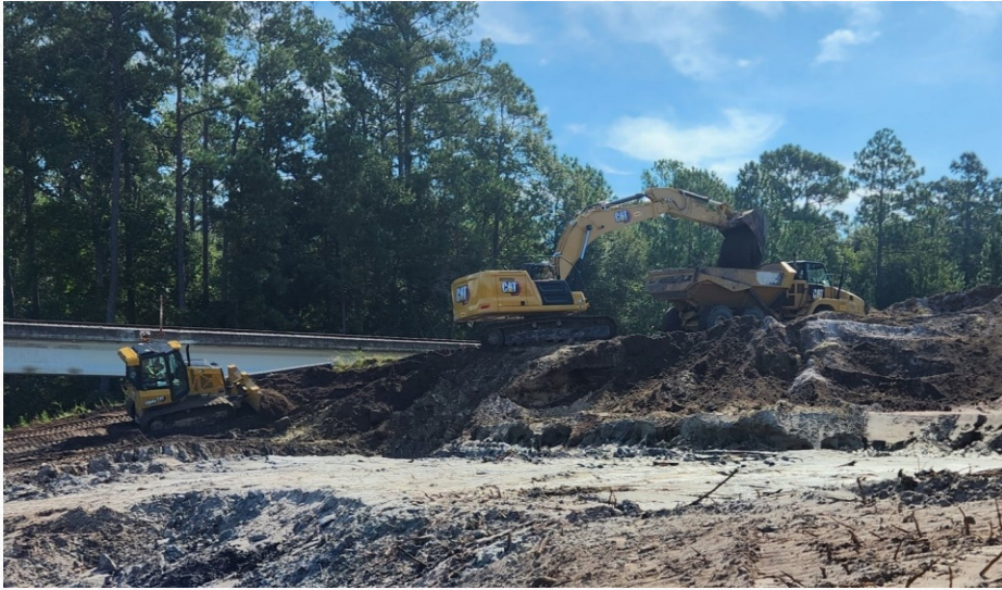
Loading Material for Coffer Dam Base
