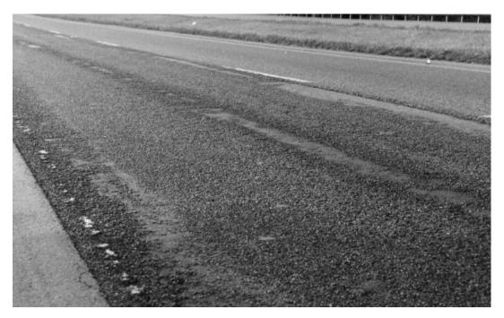
**Description**: Raveling is the wearing away of the pavement surface caused by the dislodging of aggregate particles or loss of asphalt binder. Raveling indicates either a hardening or poor application of asphalt binder.
