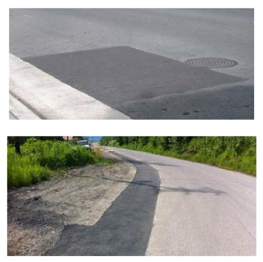
**Description:** Patching is defined as any surface area of the existing pavement that indicates some type of maintenance repair has taken place. They may be in spot locations, along one or both edges, in the wheel paths, across the entire surface for short distances, or a combination of any of these.
