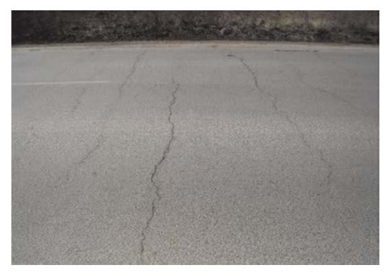
**Description:** Block cracks divide the pavement into roughly rectangular pieces. Block cracking is not load-associated. Cracks are generally caused by shrinkage of the asphalt concrete and daily temperature cycling. Wheel path loads can increase the severity of block cracking if water is allowed to penetrate into the cracks. It is therefore very important to seal these cracks to prevent water penetration into the base materials.
