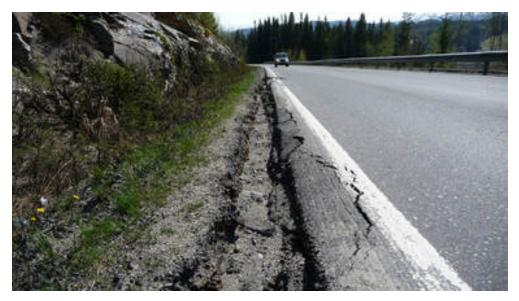
**Description:** The pavement edge is the transition where the pavement drops off vertically to the shoulder of the roadway. When the drop offs are in the range of more than 2 inches, the potential exists for a vehicles front tire to scrub against the pavement edge and not be able to return to the road surface without an abrupt and excess angle.
