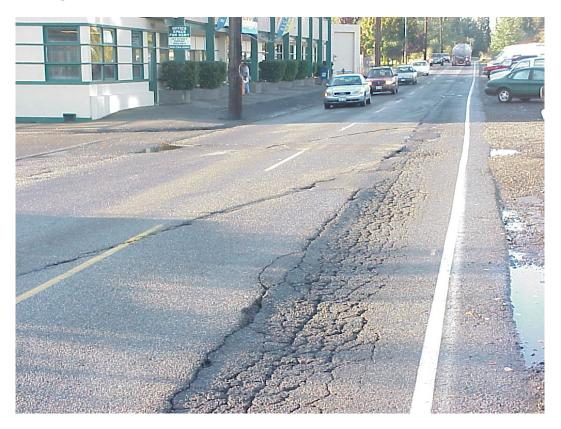
**Description:** A rut is a surface depression in the wheel path(s) or at the edge of pavement. Rutting comes from a pavement deformation in any of the pavement layers or the subgrade, usually caused by consolidation or lateral movement of the materials due to traffic loads. Movement in the mix in hot weather or inadequate compaction during construction is the main cause of rutting.
