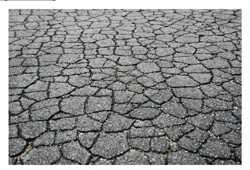
**Description:** Alligator cracking is a load-associated structural failure. The failure can be either in the surface, base, or subgrade. Alligator cracking was the most commonly observed distress in performing this assessment.
