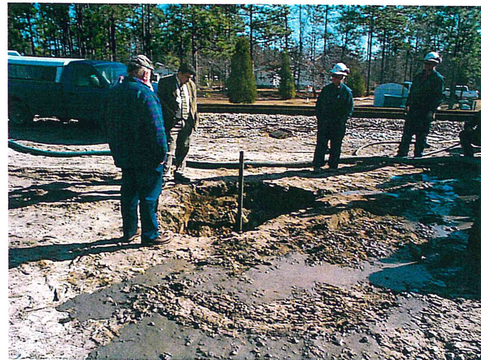
Photo 4. Sink Which Occurred Under Drill Rig at SPC-3.
