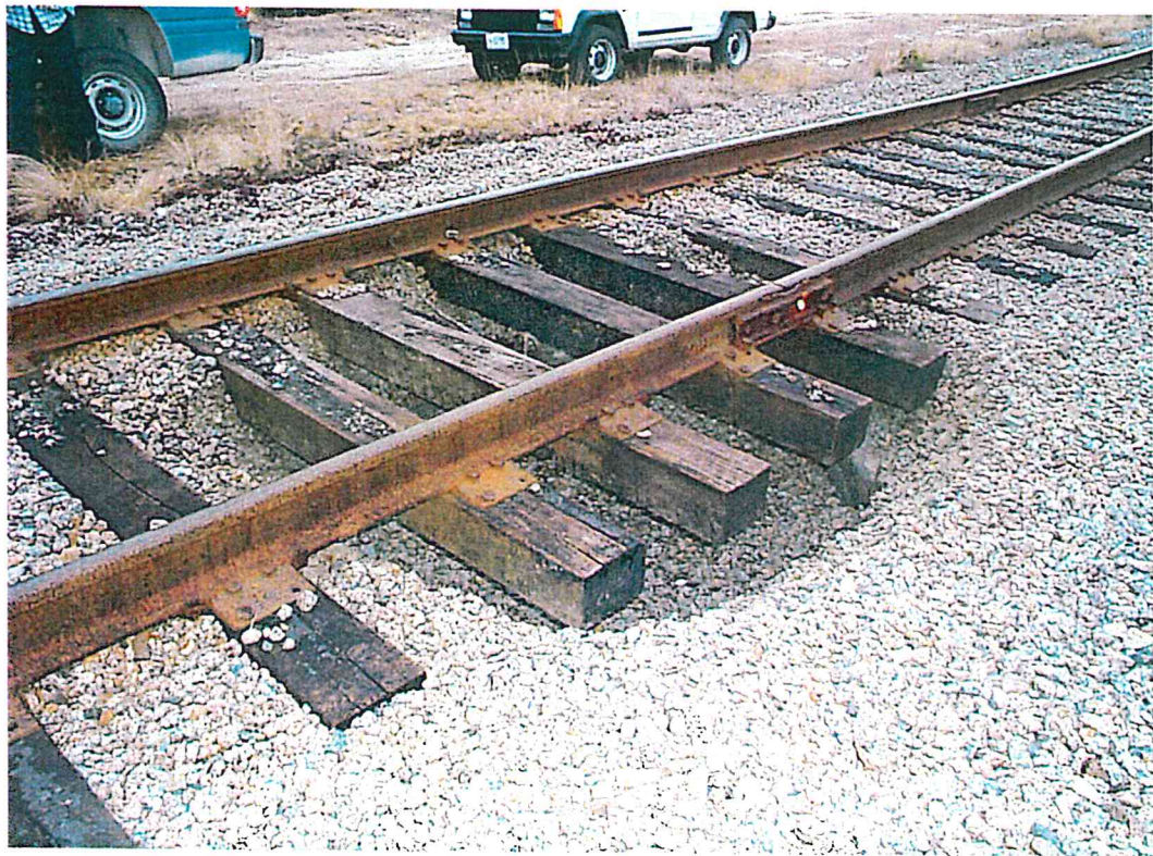
Photo 1. New Sinkhole Under Track at Station 837+77.
