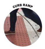
A curb ramp provides a combined ramp and landing to accomplish a change in level at a curb between the sidewalk and the street.
