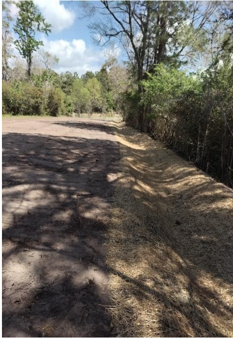
North Shore Drive Stormwater Management Swale Construction
