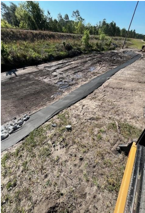
Fifty Lakes Drive Basin Slope Fabric Underlayment
