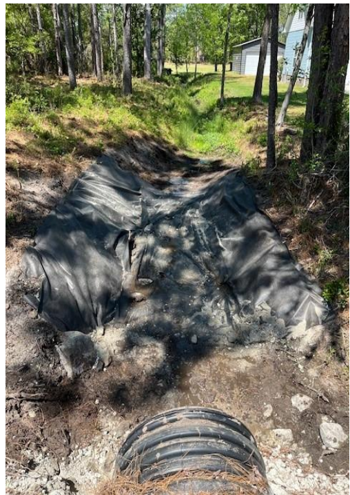
Culvert Scour Hole Repair
