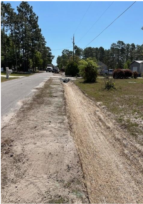
New Ditch Construction
