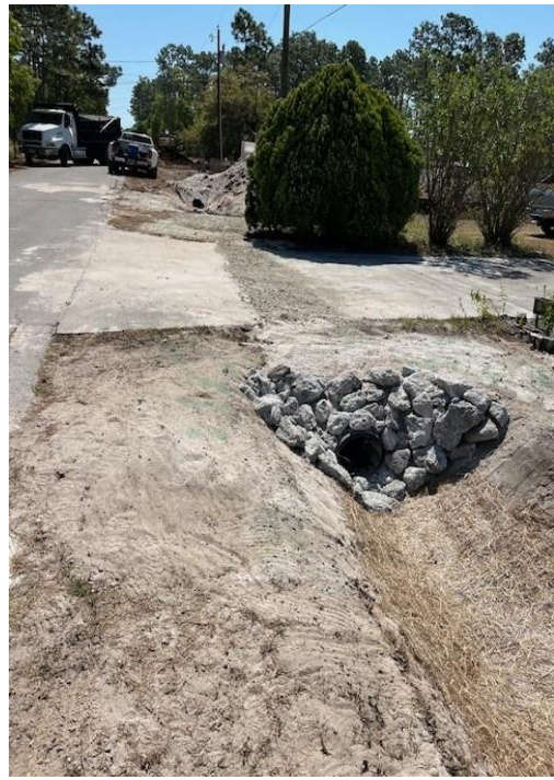
Pipe Culvert Outlet Protection
