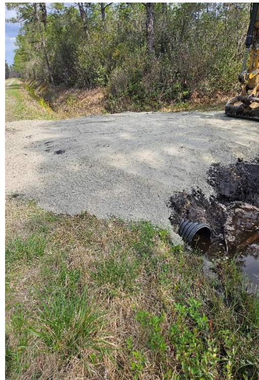
Stormwater Management Typical Pipe Replacement
