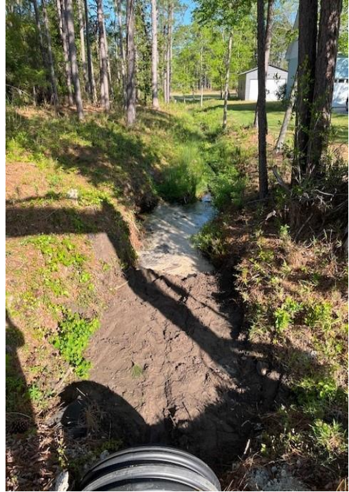
Culvert Scour Hole Repair
