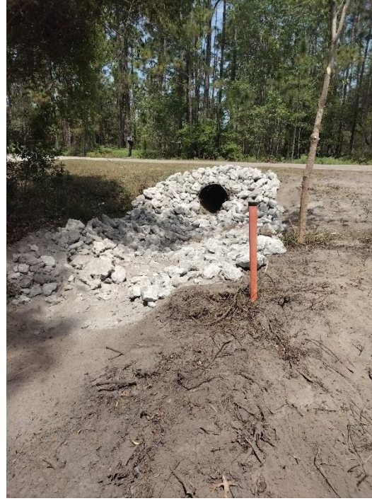
Primary Ditch Clearing (view upstream) Re-Shaping and Rip-Rap Protection
