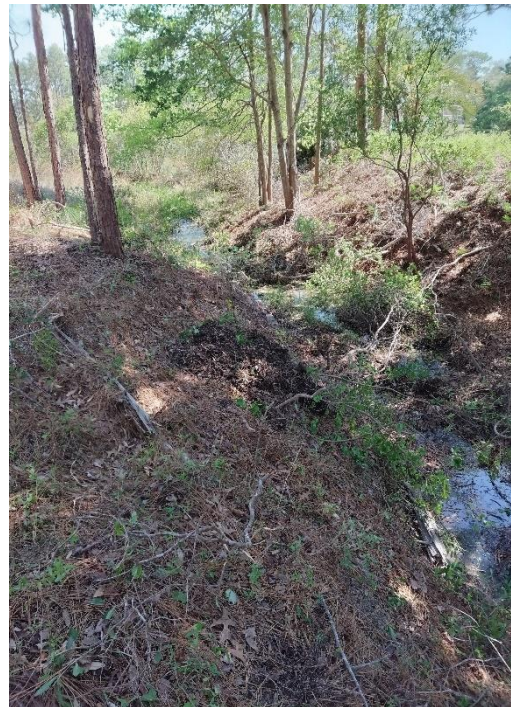
Primary Ditch Clearing and Re-Shaping
