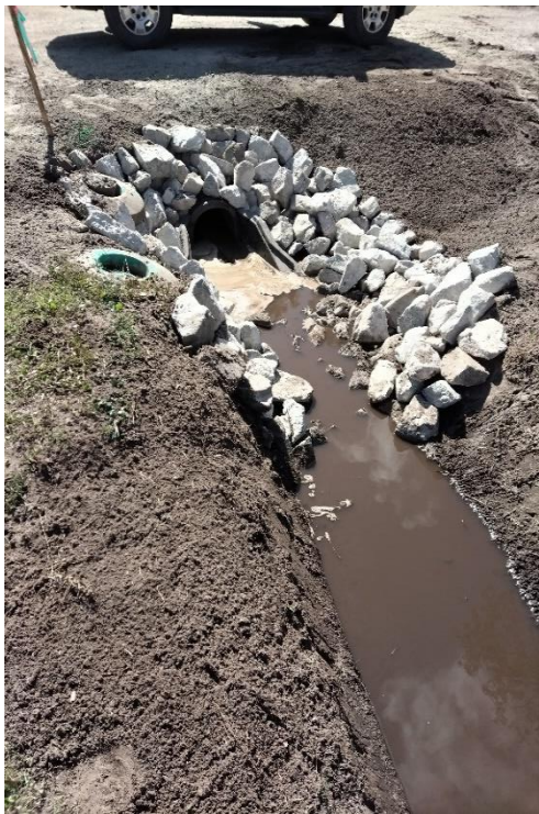
Stormwater Management General Pipe Outlet Protection
