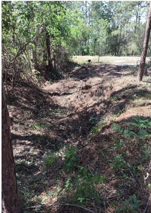
Primary Ditch Clearing and Re-Shaping
