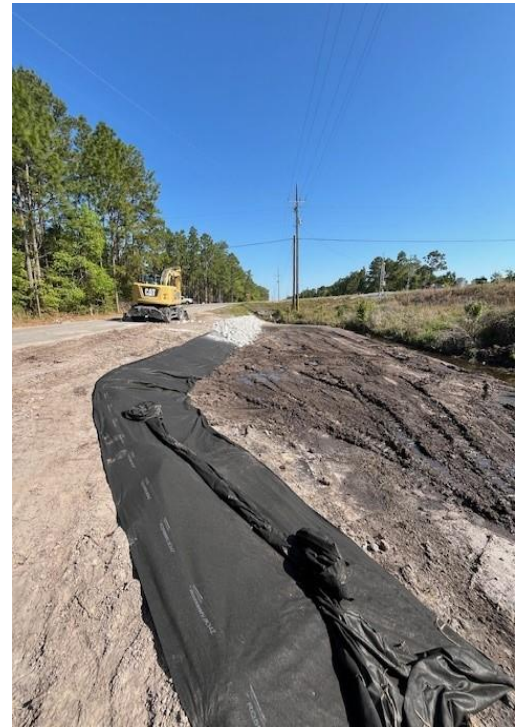
Fifty Lakes Drive Basin Slope Fabric Underlayment
