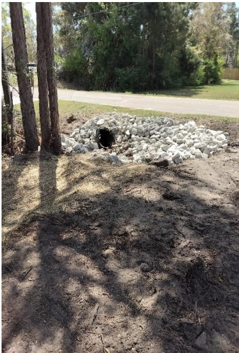
North Shore Drive Inlet Rip-Rap Protection
