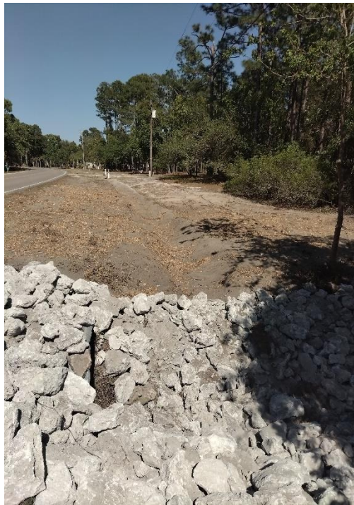
Primary Ditch Clearing Secondary Roadside Ditch Shaping
