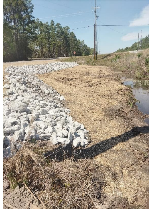
Fifty Lakes Drive Basin Completion
