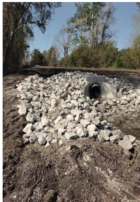
North Shore Drive Head Wall & Rip-Rap Protection
