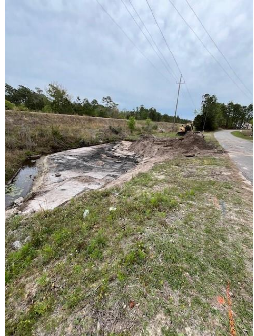
Fifty Lakes Drive Basin Excavation
