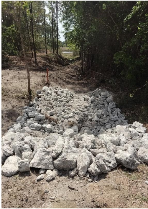
Primary Ditch Clearing (view downstream) Re-Shaping and Rip Rap Protection
