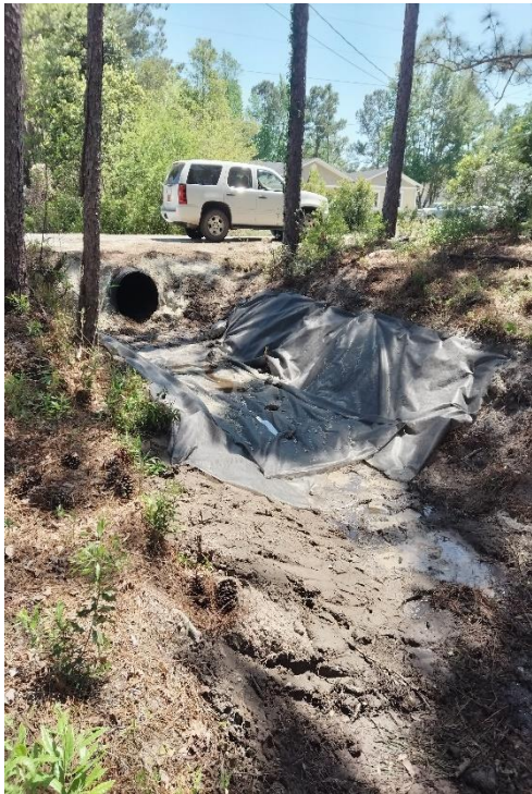
Culvert Scour Hole Repair Fabric Underlayment
