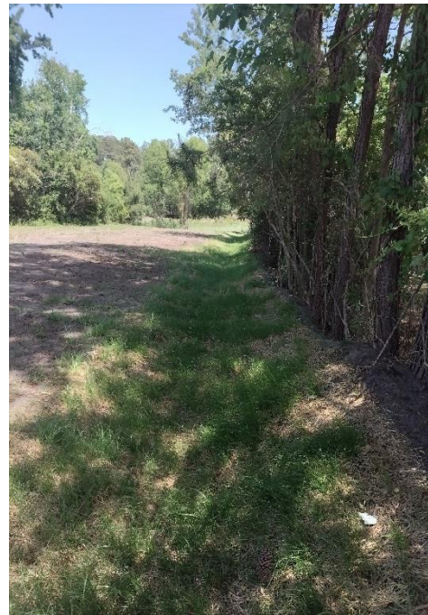
North Shore Drive Stormwater Management Stabilized Grass Swale
