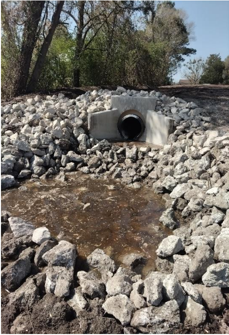
North Shore Drive Head Wall w/Plunge Pool
