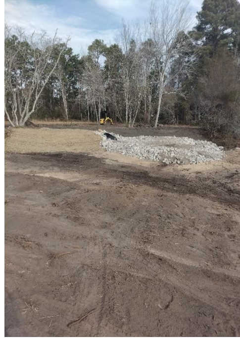
Final Grading at Pipe at Pipe Discharge
