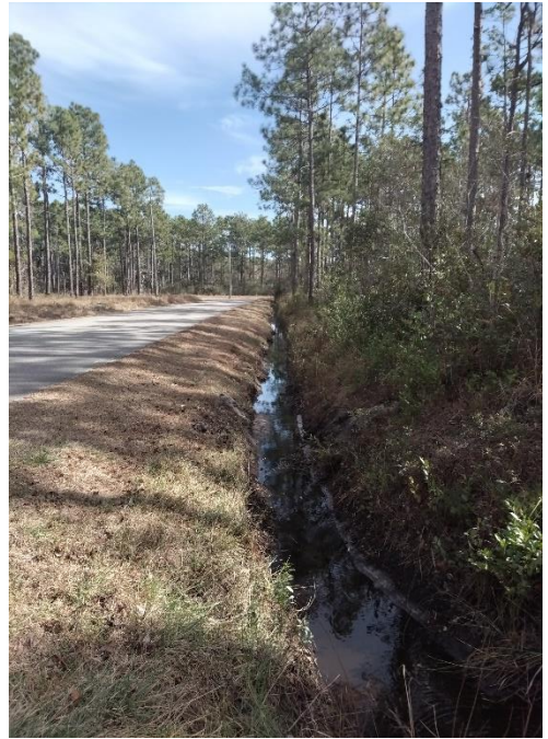
Ditch Cleaning & Reshaping Baymeade Road
