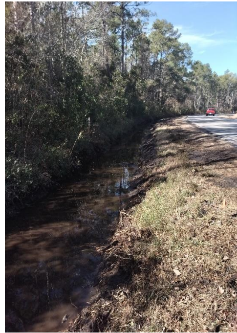
Pine Lake Rd Ditch Cleaning and Reshaping
