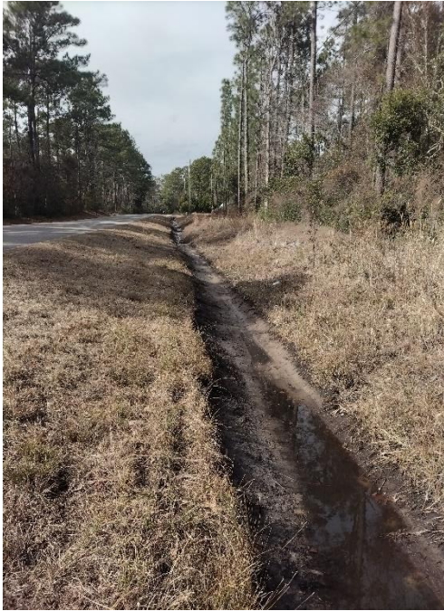
Ditch Cleaning & Reshaping Baymeade Road
