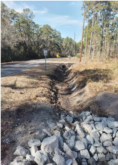
Ditch Reshaping with Rip-Rap Protection
