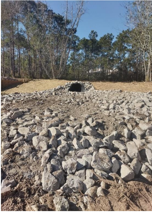
Finished Pipe Discharge w/Rip Rap Protection
