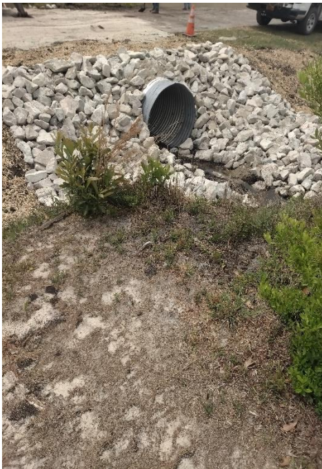
Pine Needles Road Pipe Replacement-Upstream
