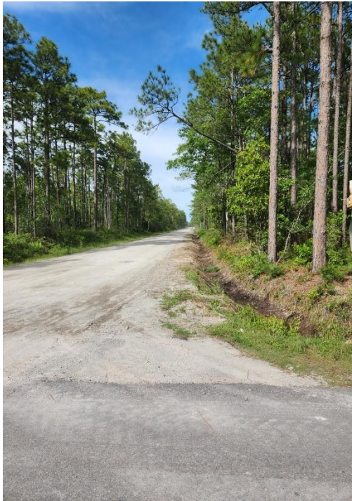
General Roadside Ditching
