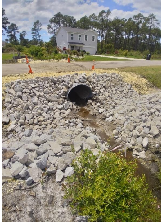
Westway Road Pipe Replacement-Upstream
