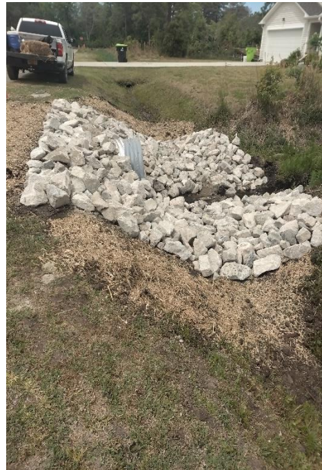
Pine Needles Road Pipe Replacement-Upstream
