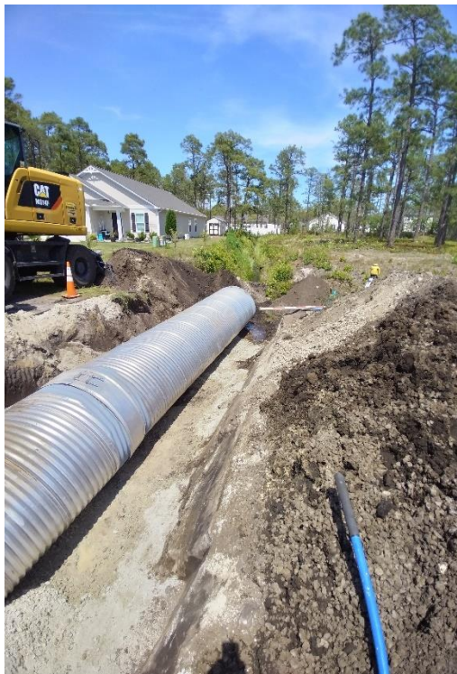
Westway Road Arch Pipe Installation
