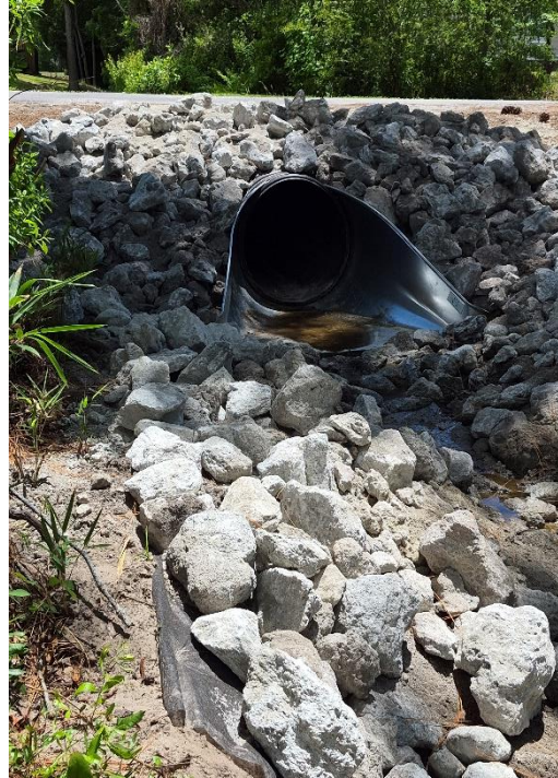
Windemere Pipe Upgrade Downstream New FES and Rip-Rap
