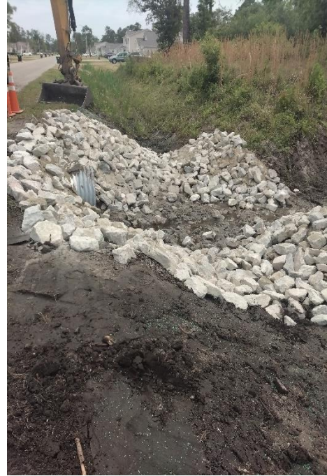
Pine Needles Road Pipe Replacement-Downstream
