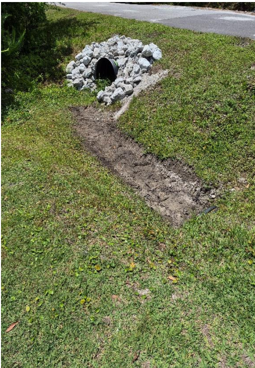
Windemere Cross Culvert Rip-Rap Protection Upstream
