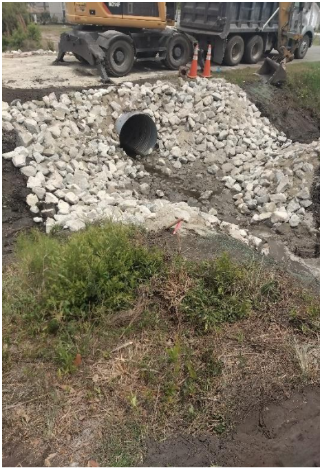
Pine Needles Road Pipe Replacement-Downstream
