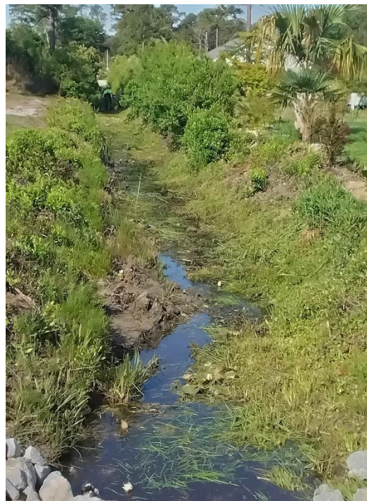
General Primary Ditch Maintenance
