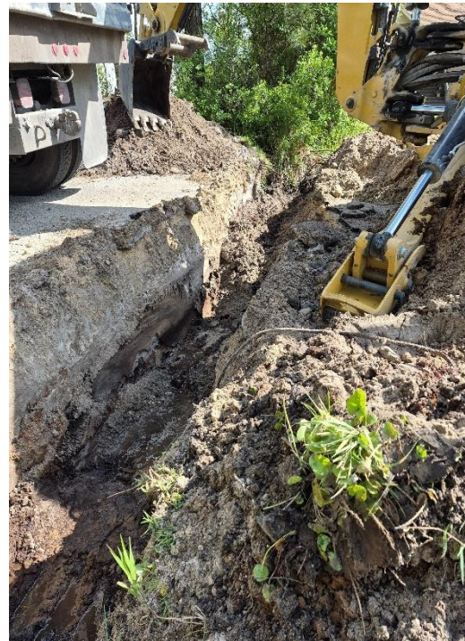
Stormwater Management Plan Pipe Excavation
