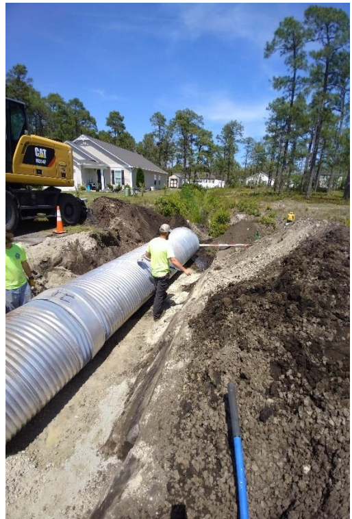
Westway Road Arch Pipe Installation
