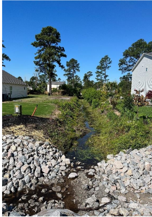
General Primary Ditch Maintenance
