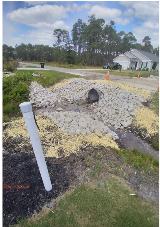
Westway Road Pipe Replacement-Downstream
