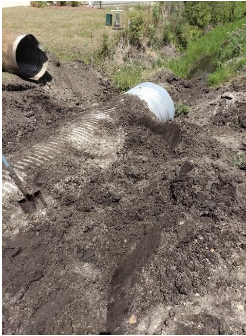
Pine Needles Road 48" CMP Pipe Installation
