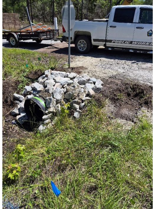
Typical Cross Culvert Repair Downstream
