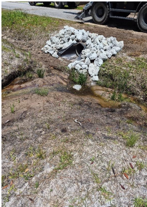
Stormwater Management Plan Pipe Replacement w/FES
