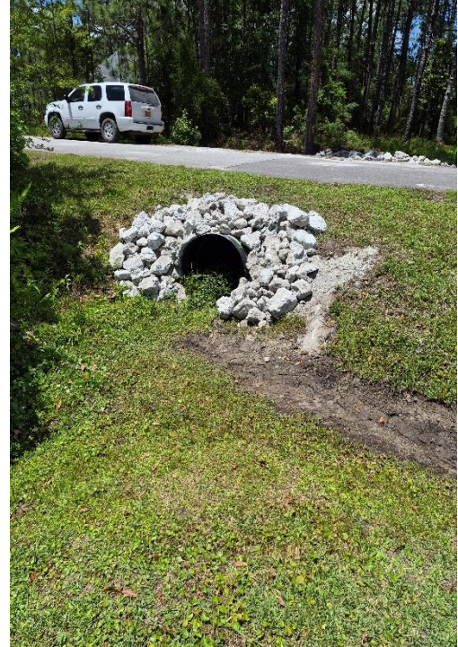
Windemere Cross Culvert Rip-Rap Protection Upstream
