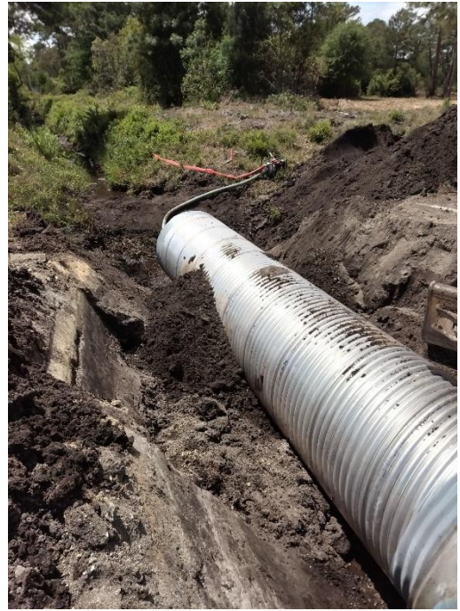
Pine Needles Road 48" CMP Pipe Installation
