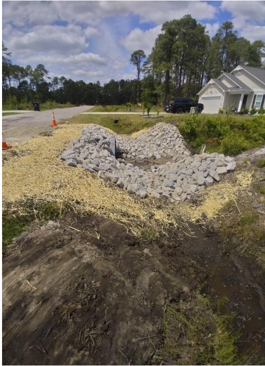
Westway Road Pipe Replacement-Upstream
