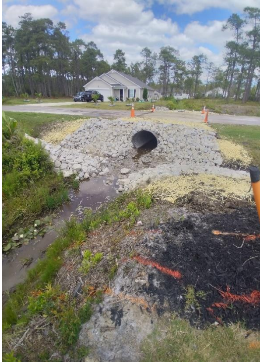
Westway Road Pipe Replacement-Downstream
