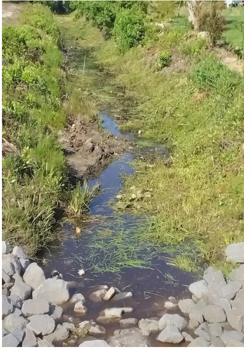
General Primary Ditch Maintenance
