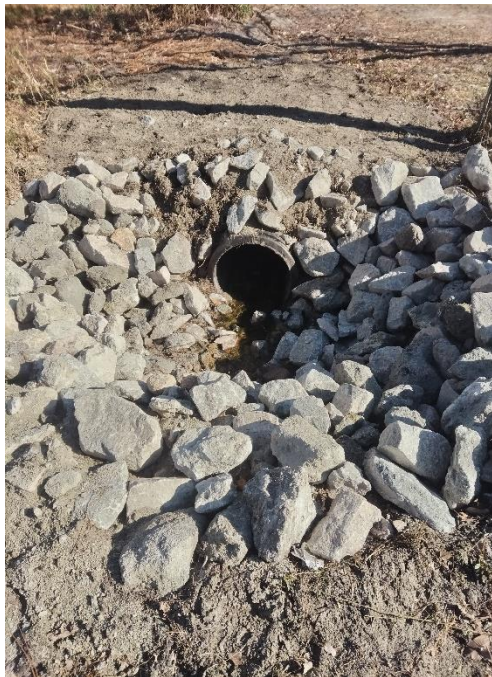
24" Intake at Pine Lake Rd And Miller Road
