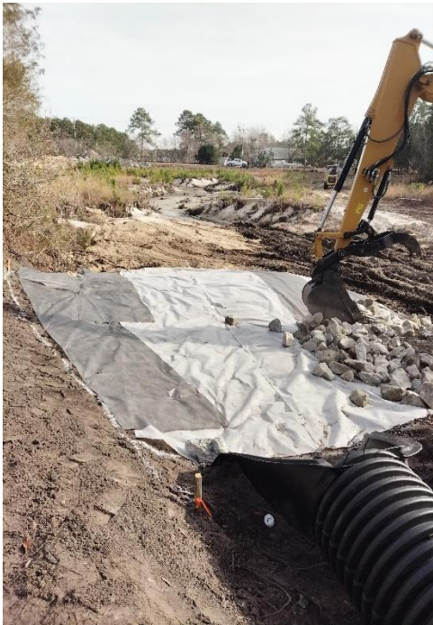
Erosion Fabric Placement at Pipe Discharge
