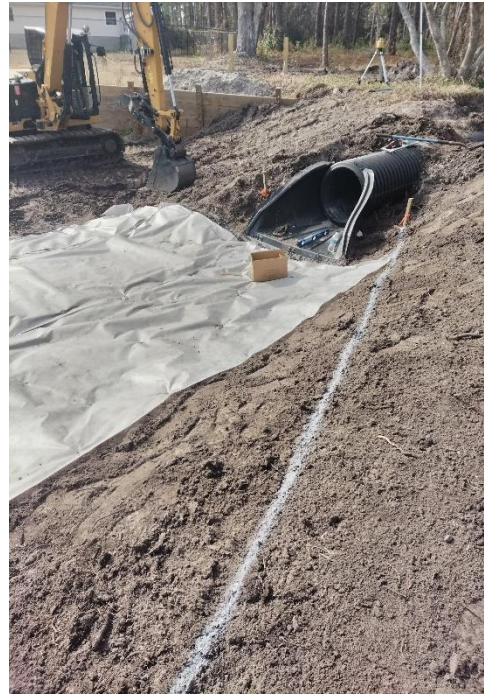
Erosion Fabric Placement at Pipe Discharge
