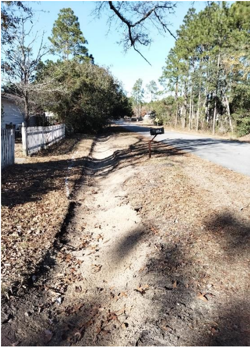
Ditch Shaping/Cleaning
