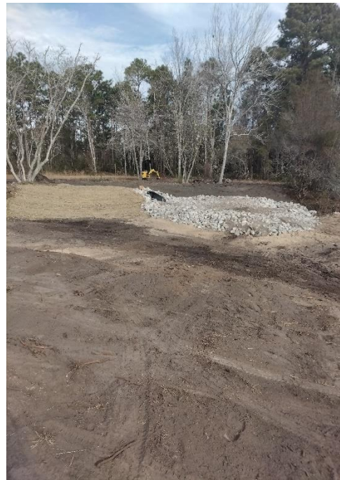
Rip-Rap Apron at Pipe Discharge
