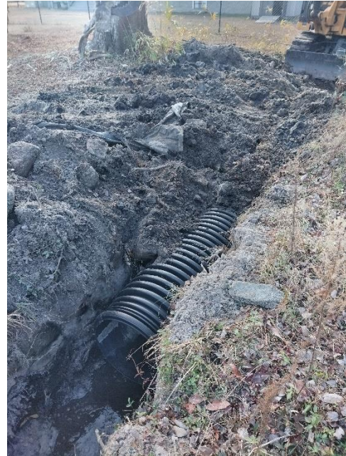
Pipe Culvert Installation
