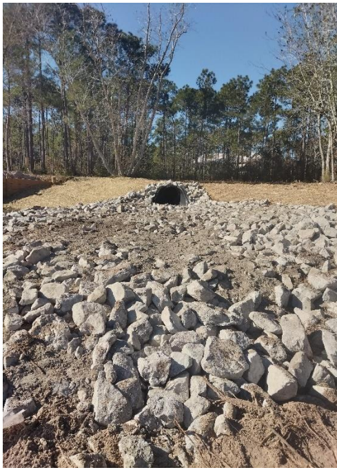
Rip-Rap Apron at Pipe Discharge
