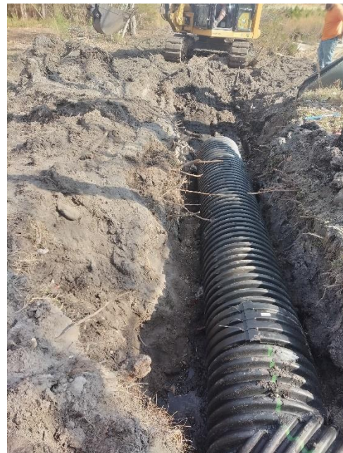
Culvert Installation
