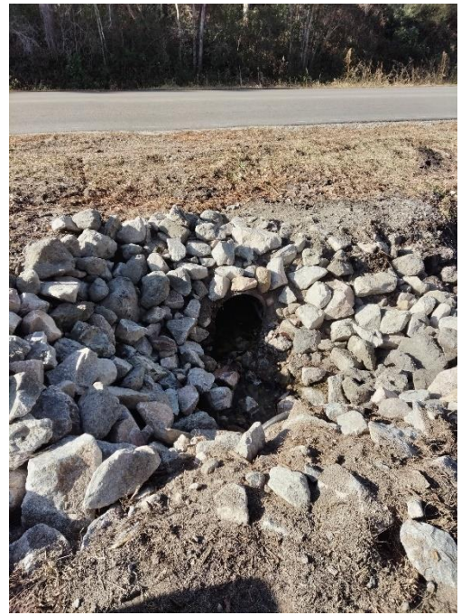
Existing 18" Pipe Rip-Rap Protection
