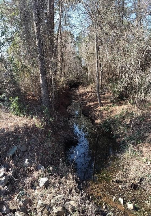
Primary Ditch Clearing And Restoration
