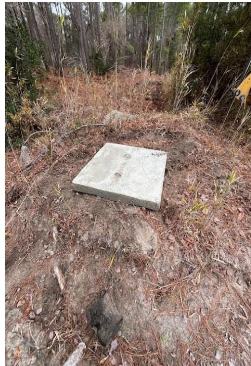
Stormwater Safety and Maintenance Repair Work
