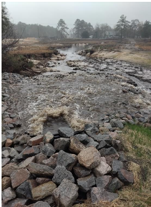
Pine Lake and Miller Rip-Rap Apron
