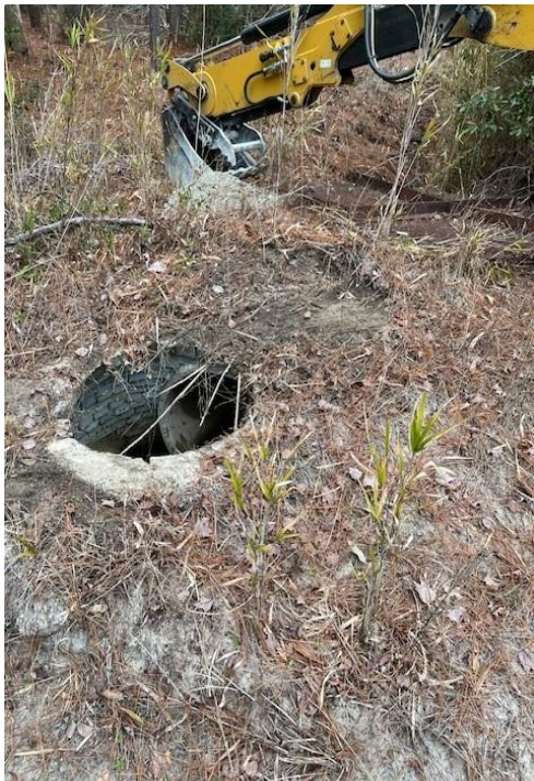
Stormwater Safety and Maintenance Repair Work
