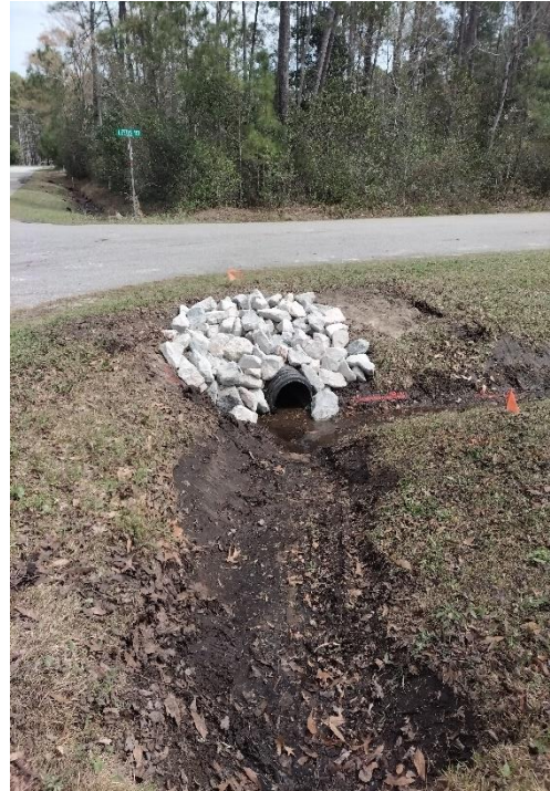
Ditch Cleaning and Reshaping With Inlet Protection
