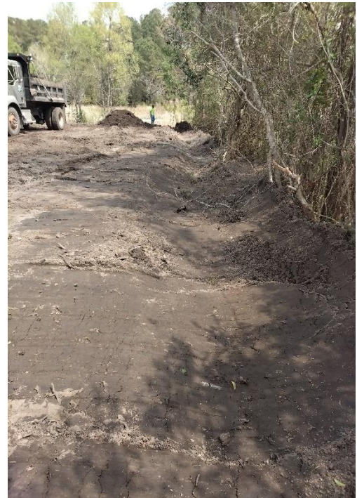
North Shore Drive Stormwater Swale Construction
