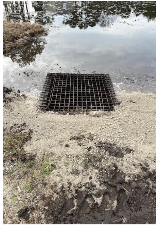
Inlet Box Maintenance & Repair
