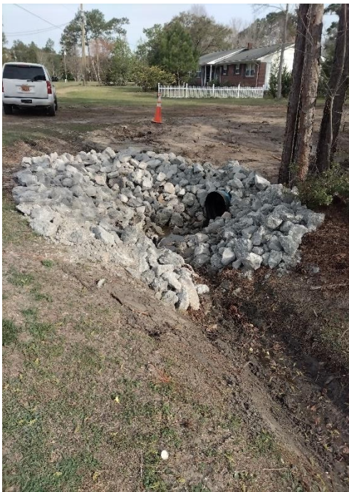
North Shore Drive Inlet Rip-Rap Protection
