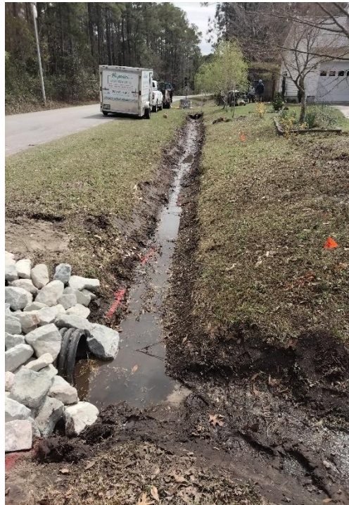
Ditch Clean and Reshaping Swale Construction
