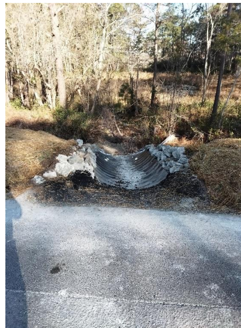
South Shore Drive Temporary Stormwater Repair
