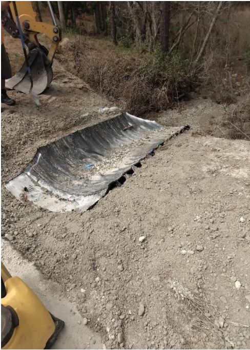
South Shore Drive Temporary Stormwater Repair
