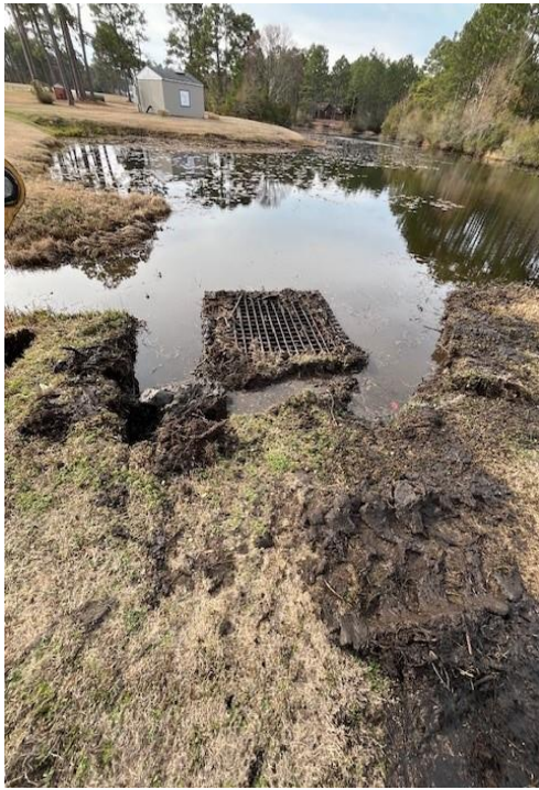
Inlet Box Maintenance & Repair
