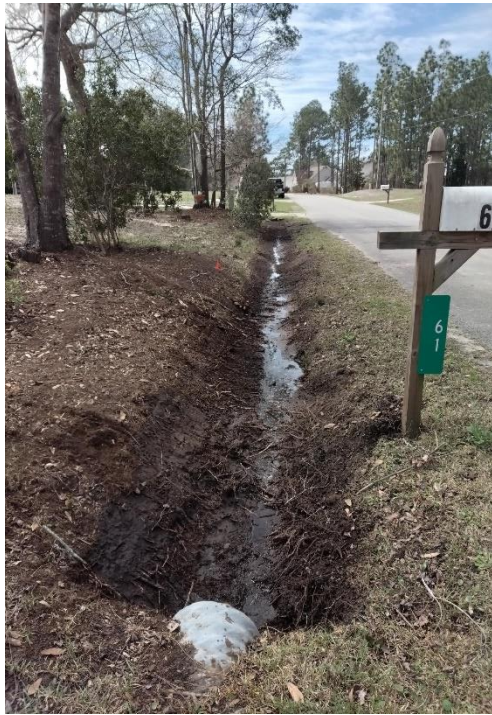
Ditch Clean and Reshaping
