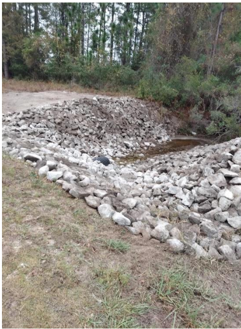
Primary Discharge with Rip Rap Protection-North Hills Drive
