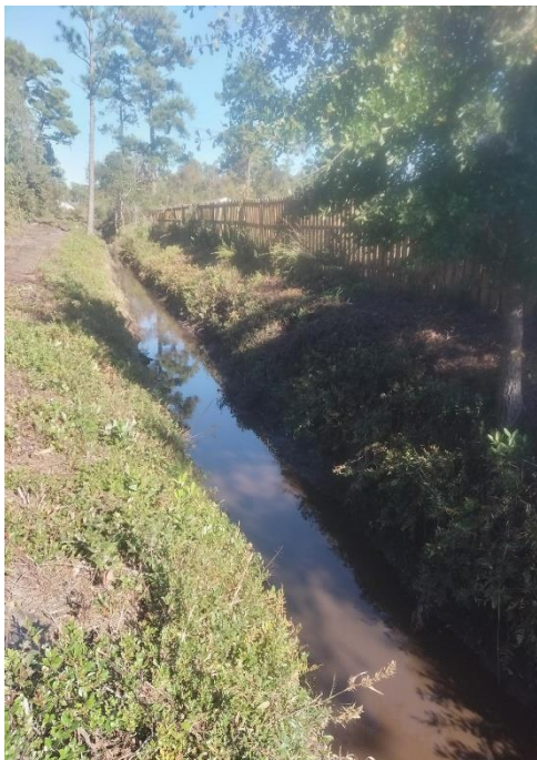
Primary ditch cleaned and groomed with maintenance path @ Gold View
