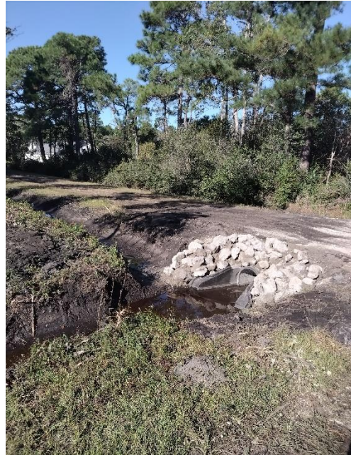
Pipe Culvert Replacement with flared end section and rip rap protection
