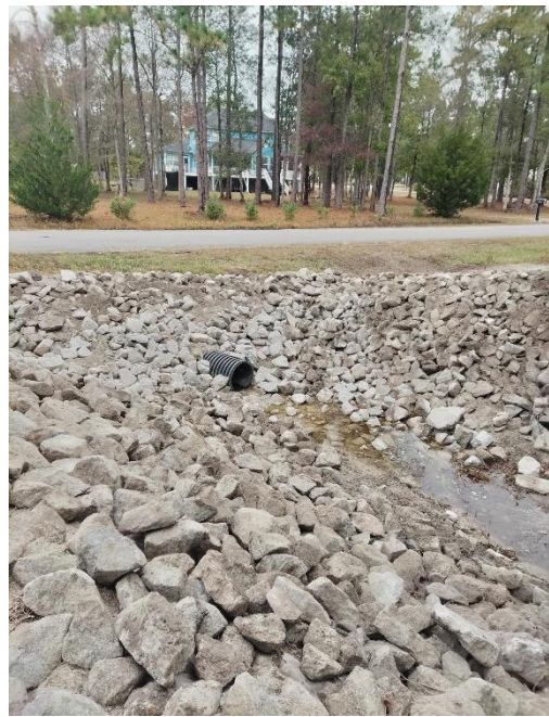
Primary Discharge with Rip Rap Protection-North Hills Drive
