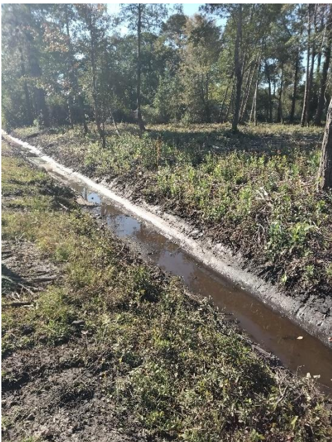
Newly reshaped and cleaned Roadside ditch
