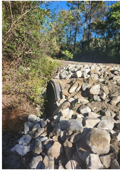
Beech Road Culvert Replacement
