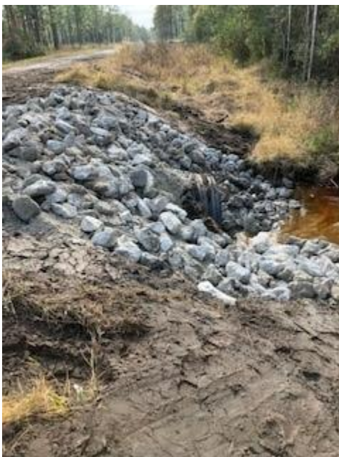
Culvert Protection West Boiling Spring Lakes Road
