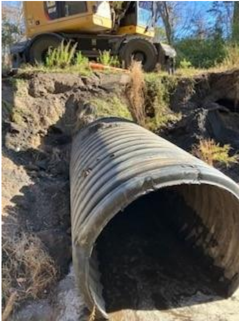
Culvert Replacement West Boiling Spring Lakes Road
