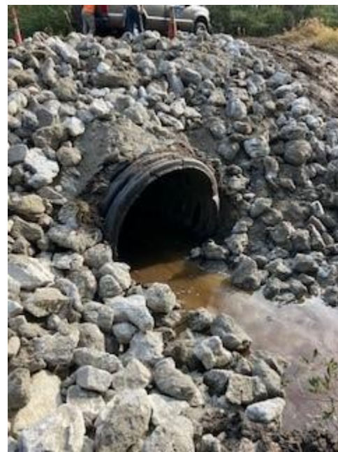
Culvert Protection West Boiling Spring Lakes Road
