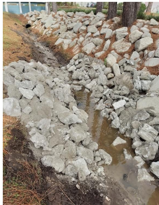
Pipe Culvert Restoration w/Rip-Rap Protection (Downstream)
