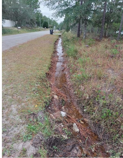
Ditch Cleaned and Shaped (typical)
