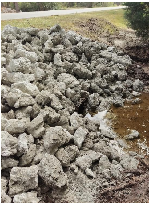
Pipe Culvert Restoration w/Rip-Rap Protection (Upstream)
